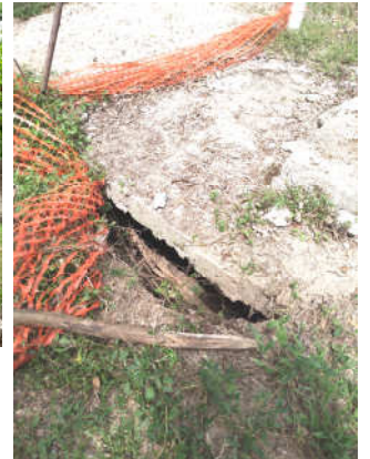
▲ Milot high school bath house the collapsed septic tank ►
