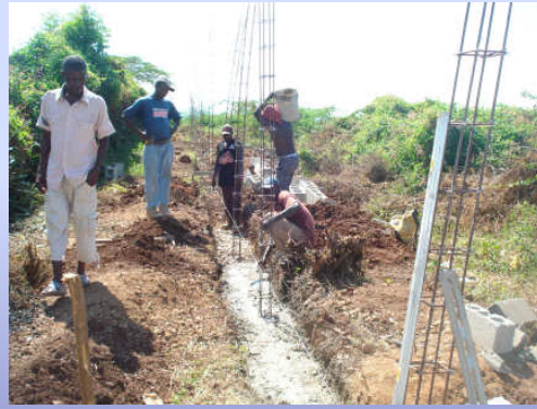
▲ Mixing & pouring concrete footer by hand The eastern side going up. ►
