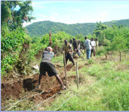
▲ Hard working Haitians digging over 1/4 mile of foundation by hand.
