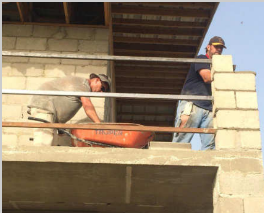
sifting sand for mortar ▲
